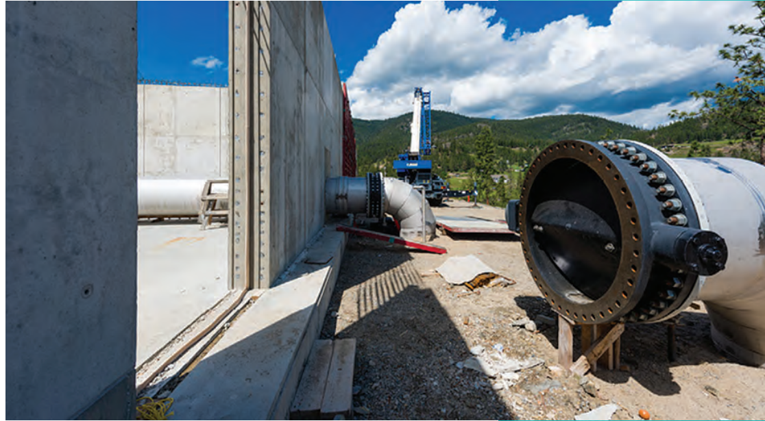
Pipe connection to the Rose Valley treated water reservoir. Credit: City of West Kelowna
